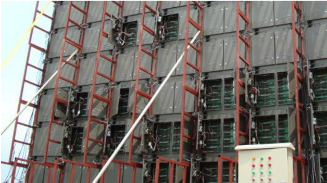
Fig.3 Connect all cables and adjust screen.
