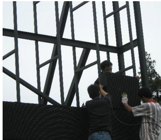
Fig.2 Experienced workers are mounting LED cabinets.
